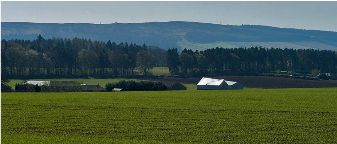
Image 5. In recognizing the roof elements as buildings in their own right the design subtly observes a characteristic of the relationship between built form and land form common to this particular landscape terrain.
