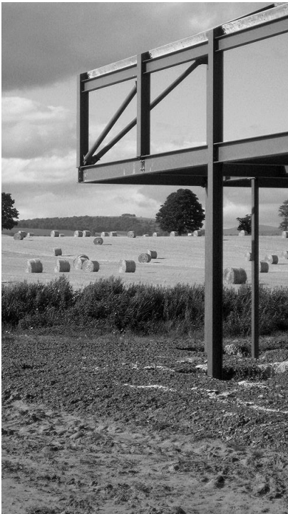
Image 9. The 3m 'erosion' created by using the attic upstand as a vierendeel truss, combines to amplify the narrative intent through building construction.
