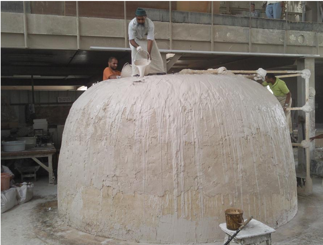
Image 14 - Initial experiments using traditional poured concrete onto formwork and a reinforcing mesh proved unworkable
